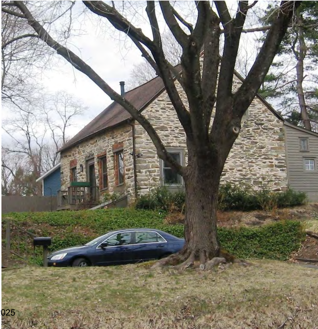
140: Frear House Wilbur Blvd Across from St John's Lutheran Church. South exit of parking lot. City of Poughkeepsie
